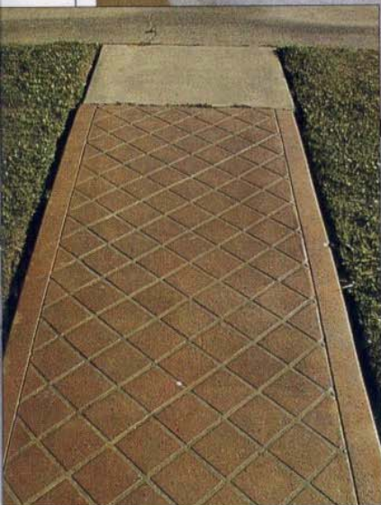
This courtyard was sprayed with Concrete Solutions' Ultra Surface Spray-Top System.
