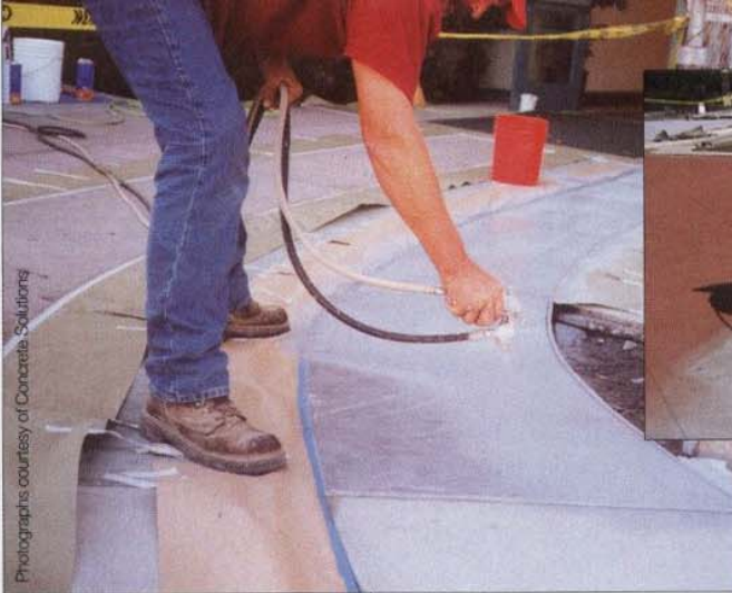
Applying the Ultra Surface Strap-Top System.
