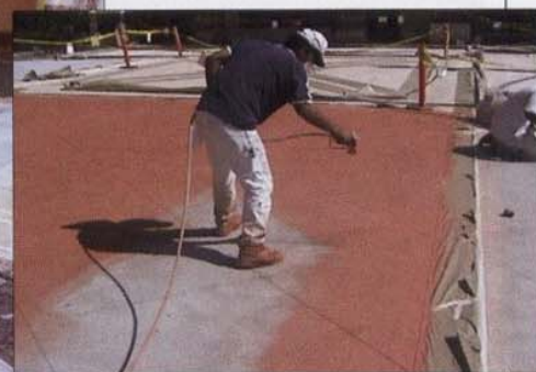
Applying the Ultra Surface Strap-Top System.
